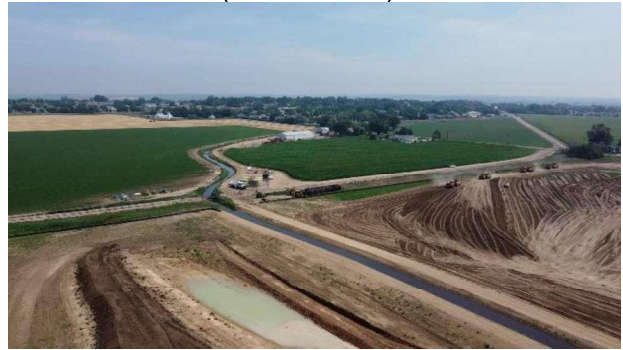
Northern end of Ditch Realignment (View: Northeast)
