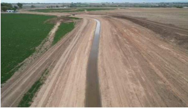
Ditch Realignment (Looking Northwest)
