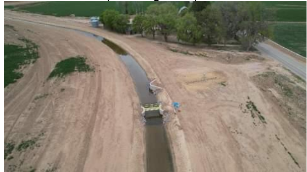
Ditch Realignment Adjacent to Telep Ave. (Looking North)
