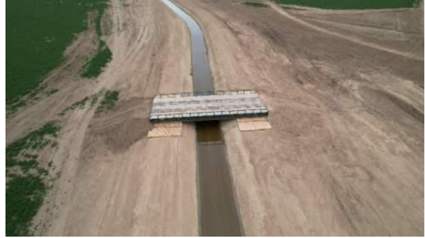
Temporary Bridge over Ditch Realignment
