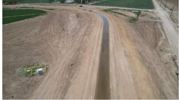
Ditch Realignment Adjacent to CR 46 (Looking East)
