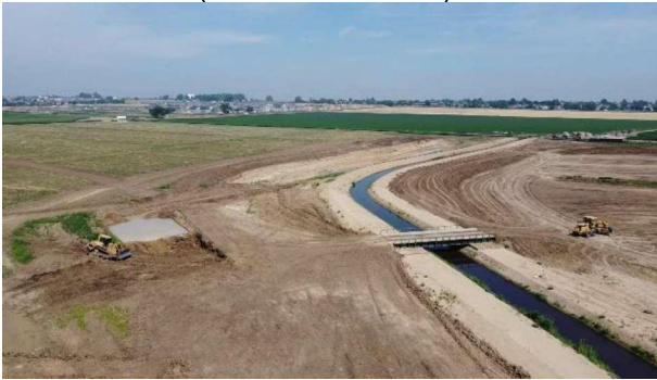
Ditch Realignment southwest of bridge (Looking Northwest)
