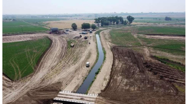
Ditch Realignment northeast of bridge (View: South)
