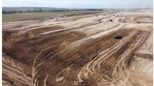
Mass Grading on site (View: Southwest)
