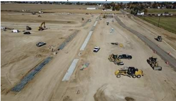
Muturu Road (View: North)
