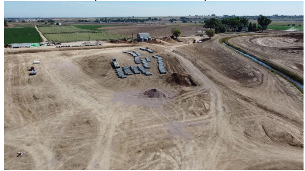
Northern end of Ditch Realignment (View: Southeast)
