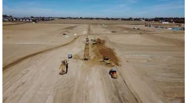
Galloway Drive Utility Improvements (View: North)
