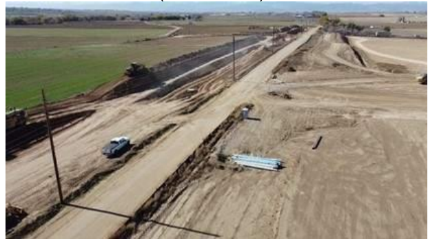
County Road 46 Waterline Improvements (View: Southwest)
