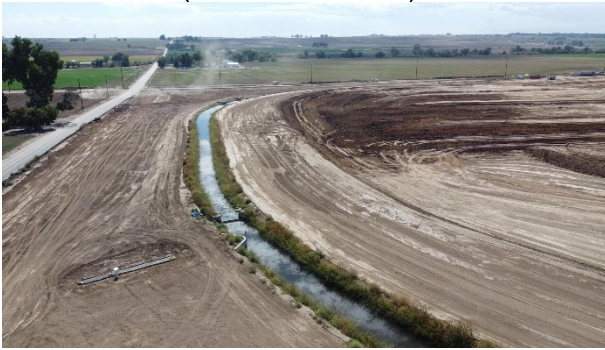
Ditch Realignment southeast of bridge (View: South)
