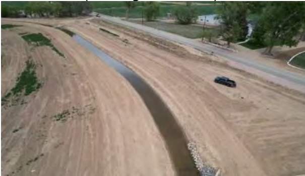
Ditch Realignment Adjacent to Telep Ave. (Looking Northeast)
