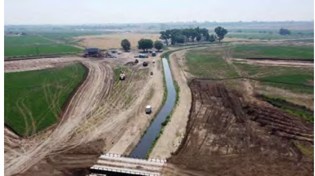
Ditch Realignment northeast of bridge (View: South)
