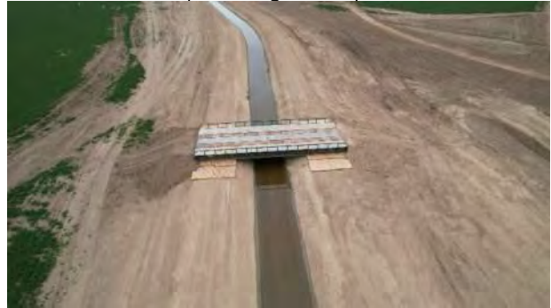
Temporary Bridge over Ditch Realignment
