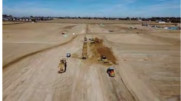
Galloway Drive Utility Improvements (View: North)
