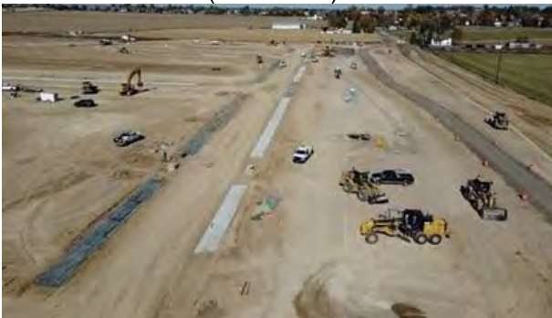
Muturu Road (View: North)
