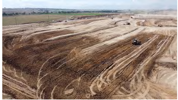
Mass Grading on site (View: Southwest)
