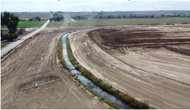
Ditch Realignment southeast of bridge (View: South)
