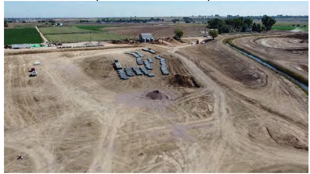
Northern end of Ditch Realignment (View: Southeast)
