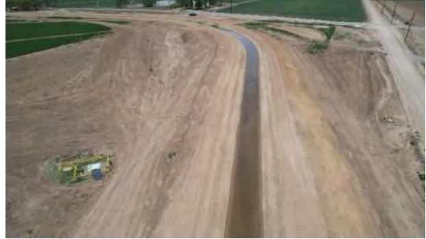
Ditch Realignment Adjacent to CR 46 (Looking East)
