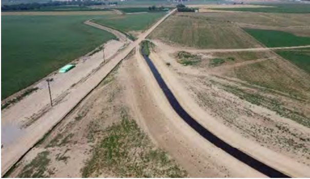
Southern End of Ditch Realignment at CR 46 (View: Southwest)
