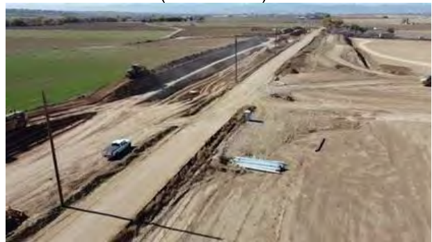
County Road 46 Waterline Improvements (View: Southwest)
