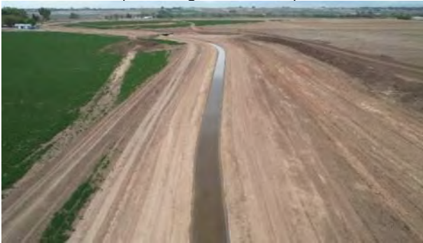
Ditch Realignment (Looking Northwest)
