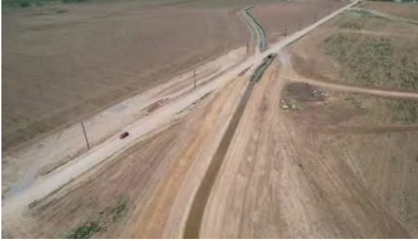
Southern End of Ditch Realignment at CR 46 (Looking Southwest)
