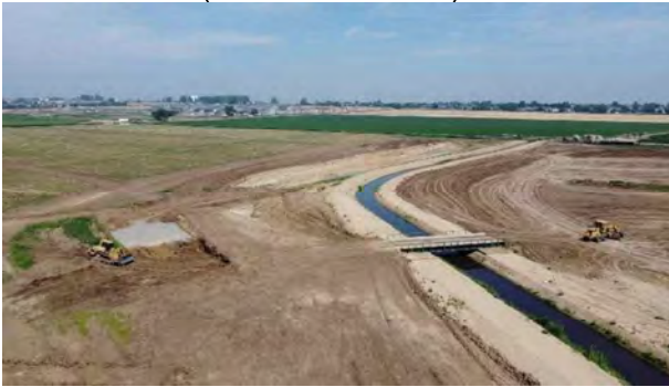
Ditch Realignment southwest of bridge (Looking Northwest)
